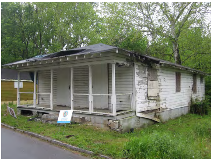
Houses currently occupying the site are in a state of distress and abandonment.
