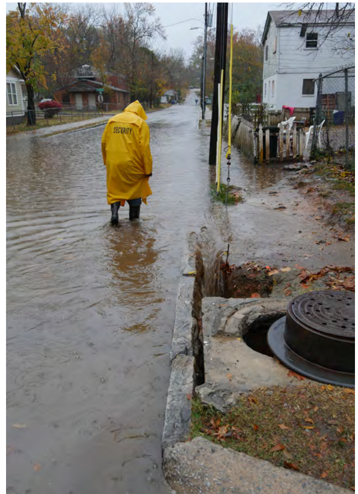
Flooding occurs on Proctor Street, just north of the park, even during relatively common rain events.
