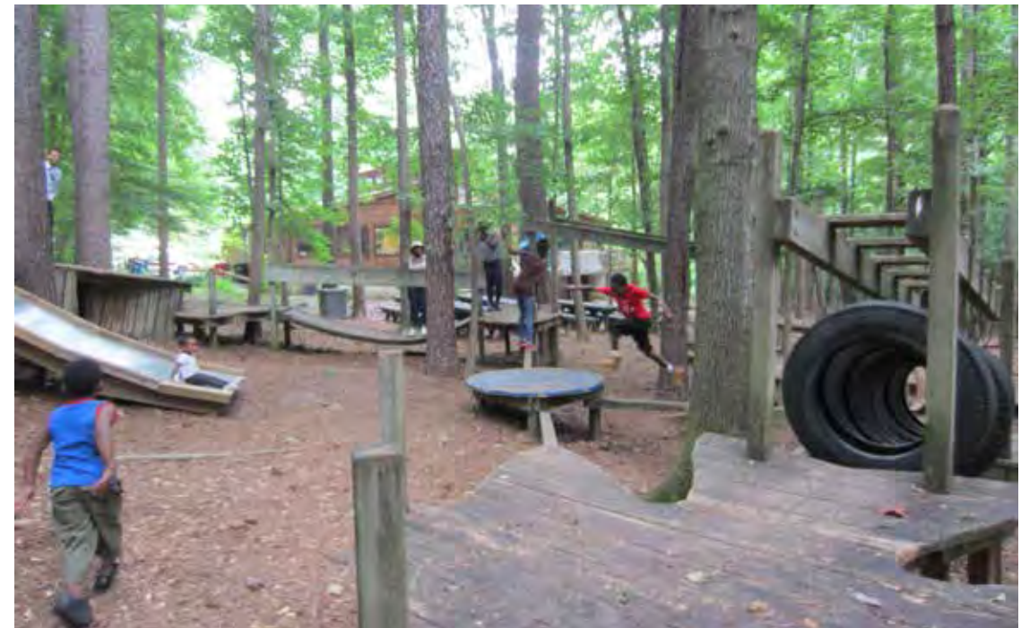
Existing Conditions of the Outdoor Activity Center Play Structure
