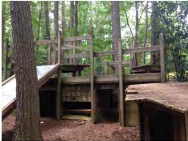
Existing Play Structure
