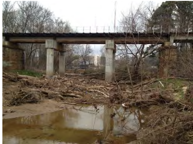
The CSX Railroad crosses the creek and proposed trail.
