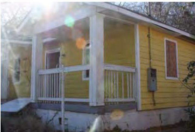
Another abandoned house that blights the community
