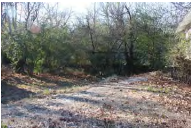
Combined sewer is partially above ground level
