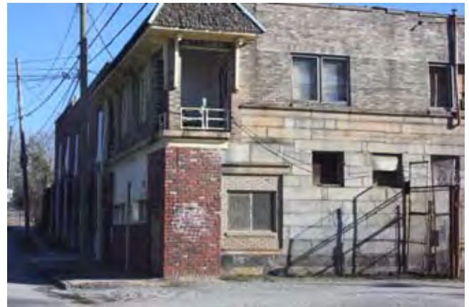
Abandoned retail building
