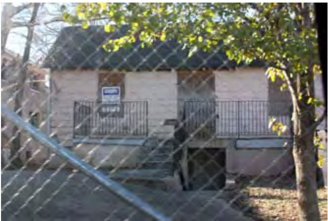
Boarded up houses are far too common in study area
