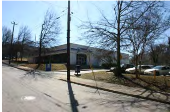
The post office which is proposed to be moved to higher ground
