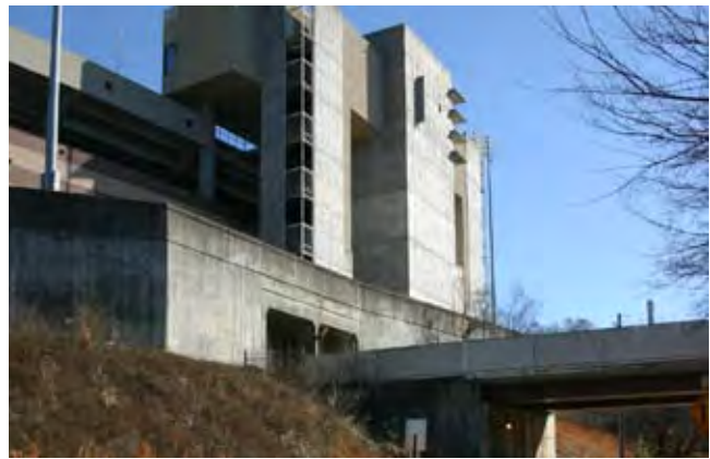
Morris Brown Stadium and the MARTA tracks that are adjacent to the proposed Sunset Avenue Park
