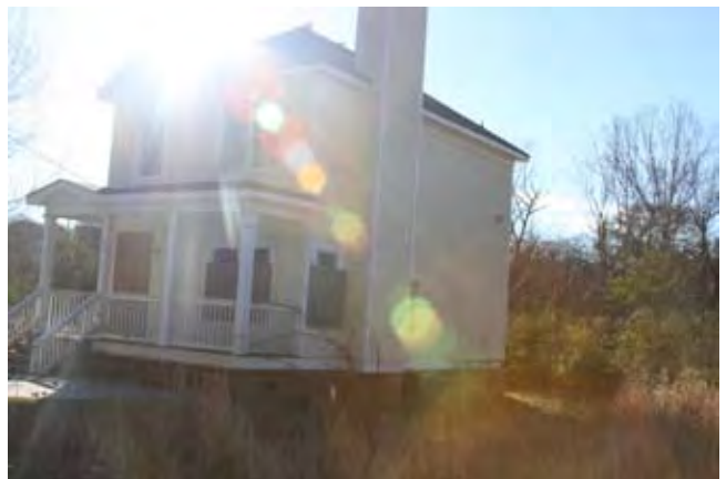
Another abandoned new house on a nearly vacant block
