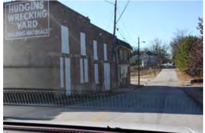
Example of existing conditions
