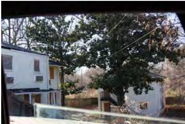
Houses in areas that flood frequently are predominantly abandoned
