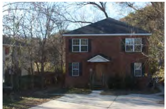
Many vacant houses such as this one were built in flood-prone areas
